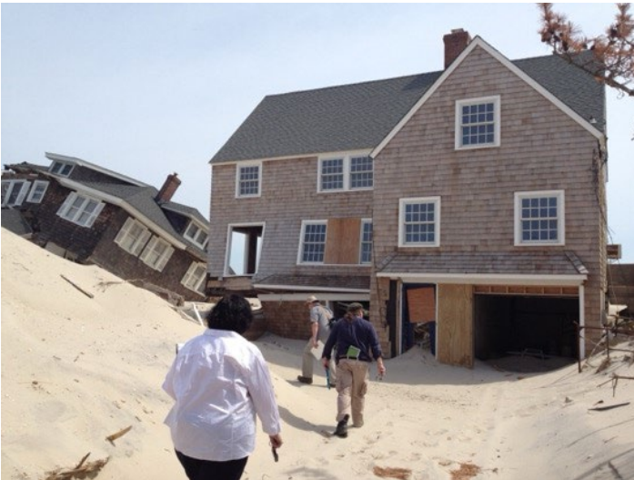
SHPO and FEMA staff survey damage after Hurricane Sandy. Courtesy of New Jersey SHPO
