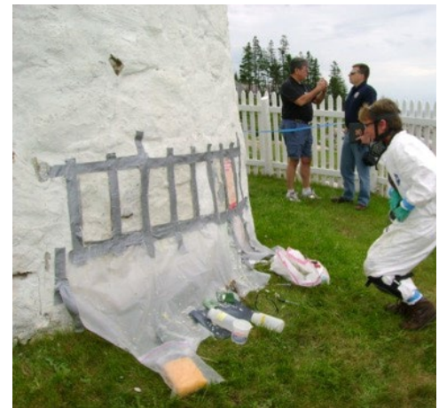
Reviewing preservation treatments at Pemaquid Lighthouse, Maine. Courtesy of Maine SHPO
